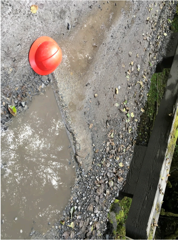
End of girder, right bank
