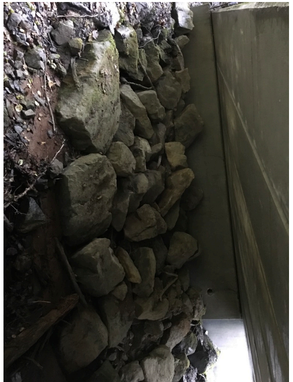
Left Bank Abutment when facing downstream
