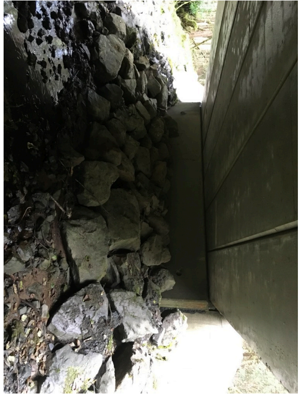
Right Bank Abutment when facing downstream
